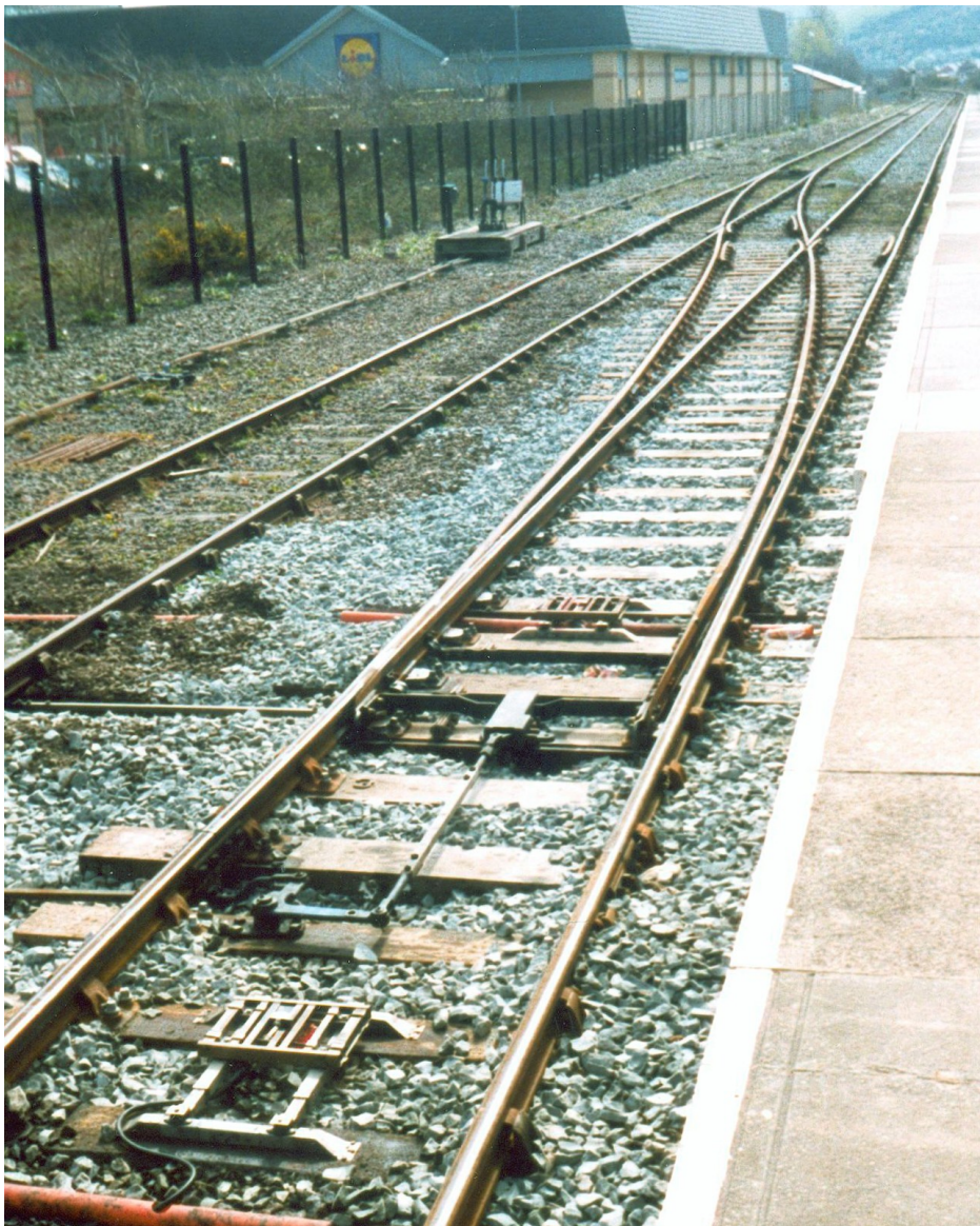
The points at Aberystwyth after repair—in time for the visit of the Black 5.
